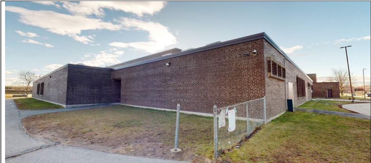
View of northeast corner of building, looking southwest.
