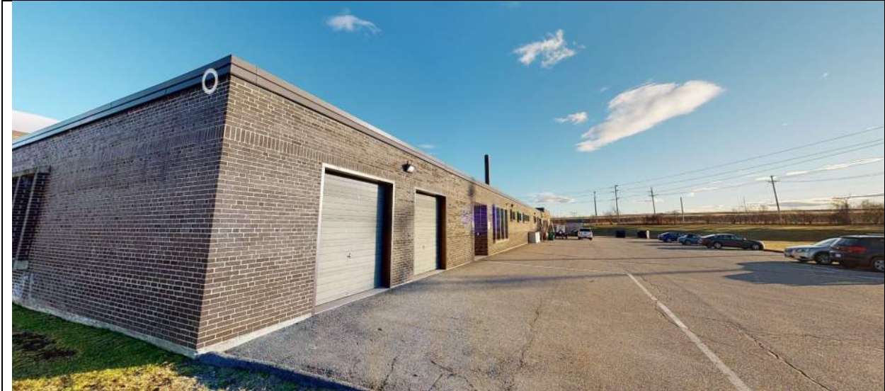
View of northwest corner of the building, looking south.
