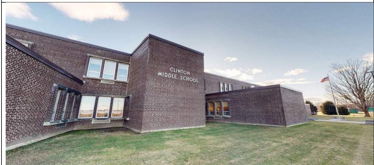
View of north side of building.
