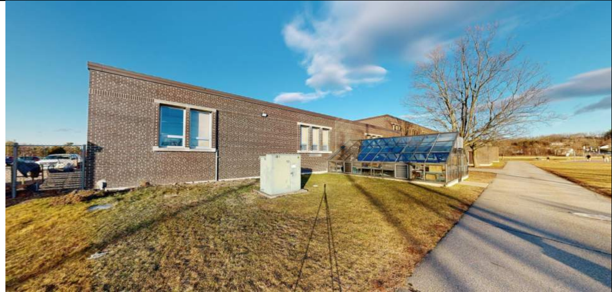
View of south side of building, showing the greenhouse, looking northeast.
