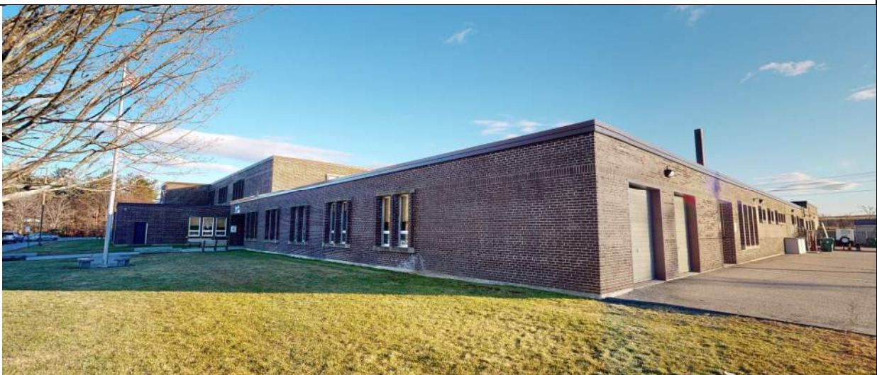
View of northwest corner, looking southeast.
