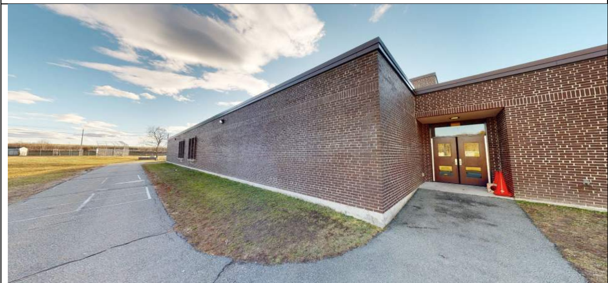
View of east side of building, looking southwest.
