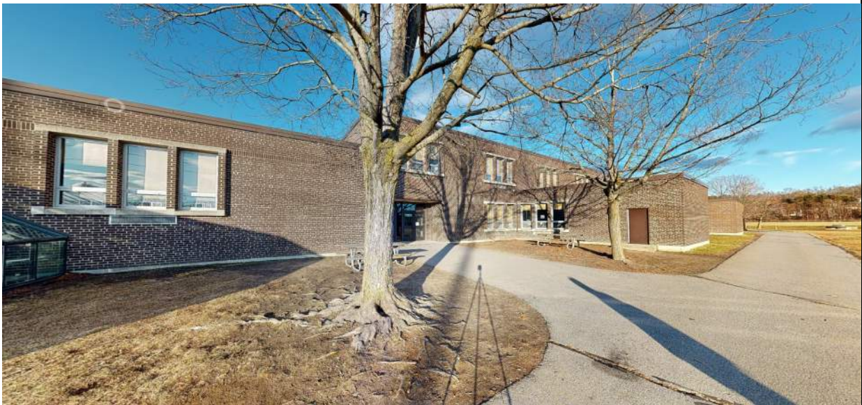
View of south side main entrance, looking northeast.
