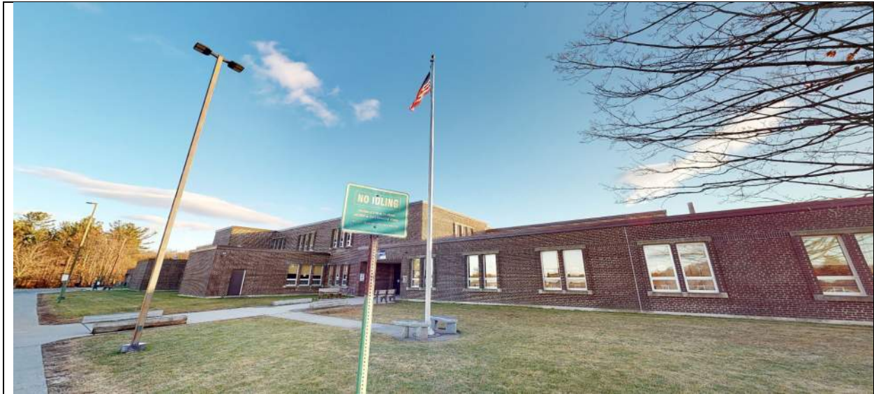
View of north side of building, looking southeast.
