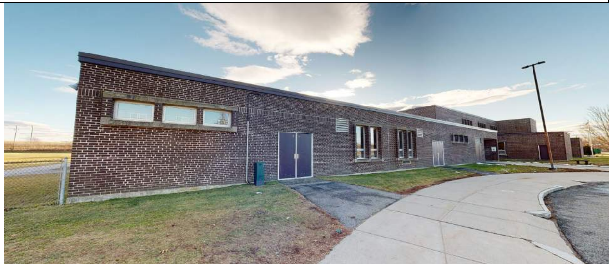
View of north side of building, looking southwest.
