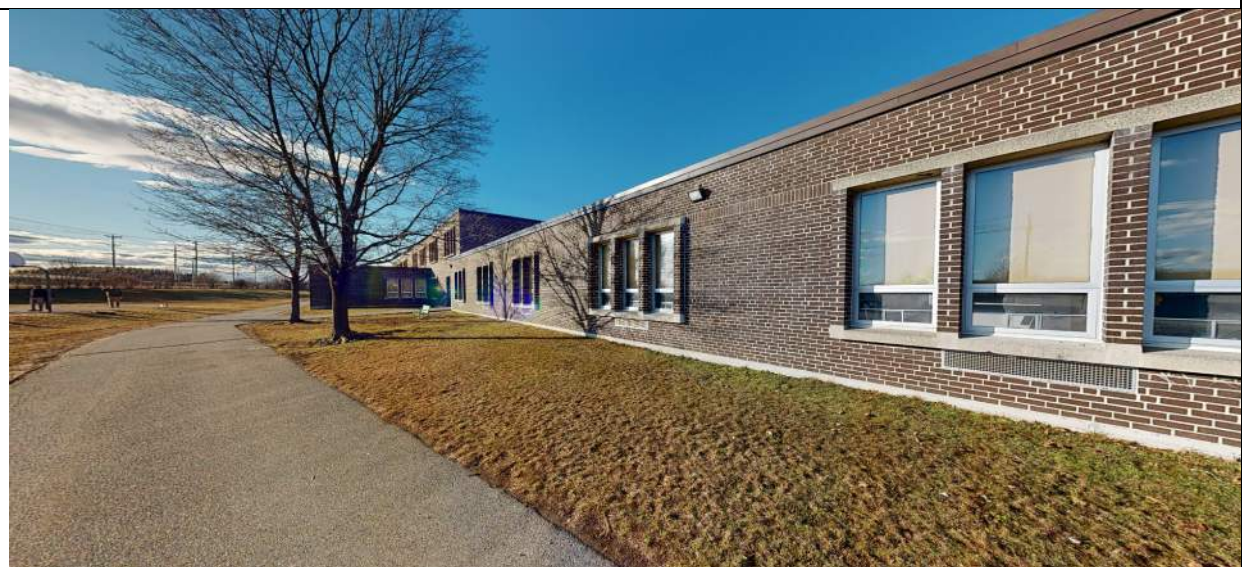
View of the southeast corner of the building, looking northwest.
