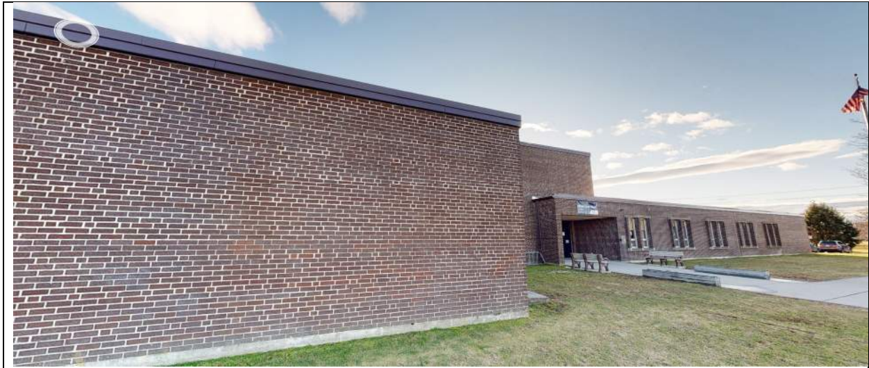
View of main entrance on north side of building.
