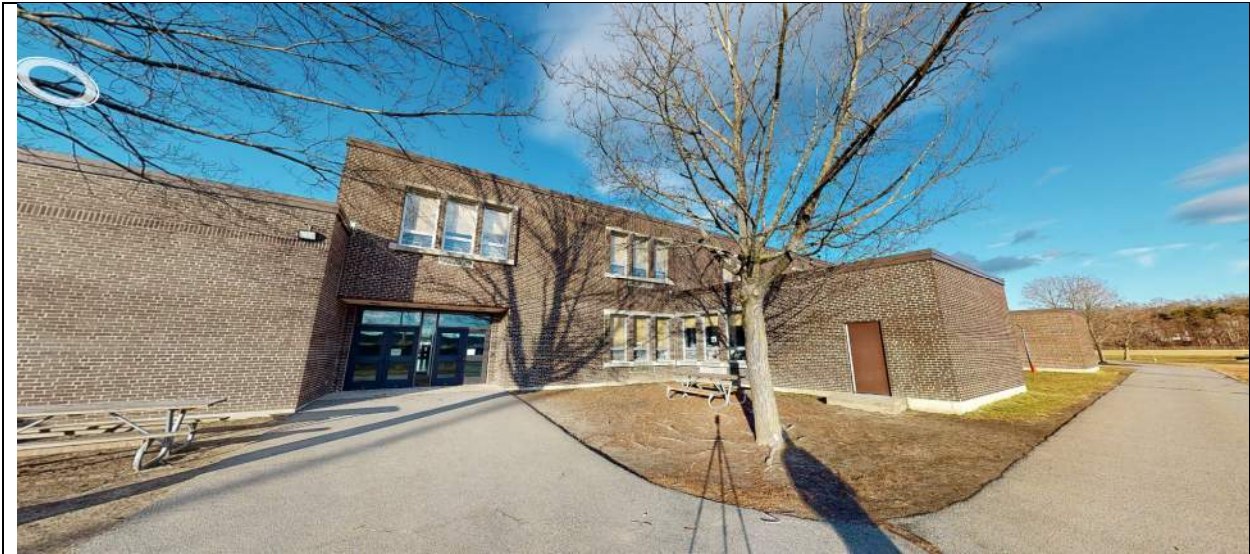
View of south side main entrance, looking northeast.
