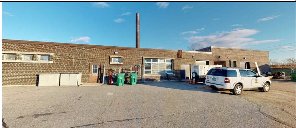
View of west side of building, looking east.
