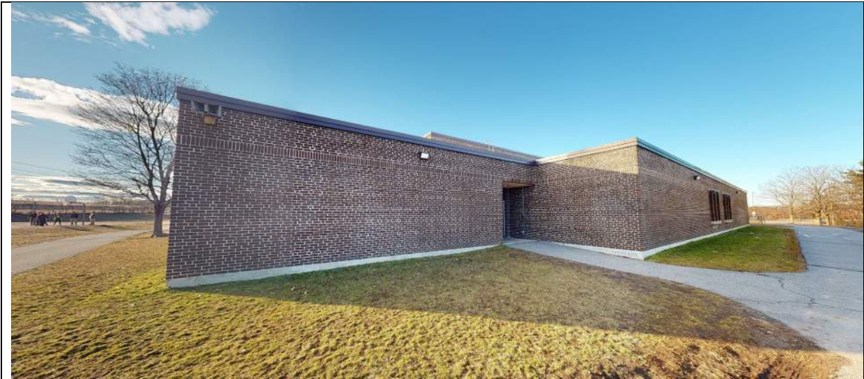
View of east side of building, looking northwest.
