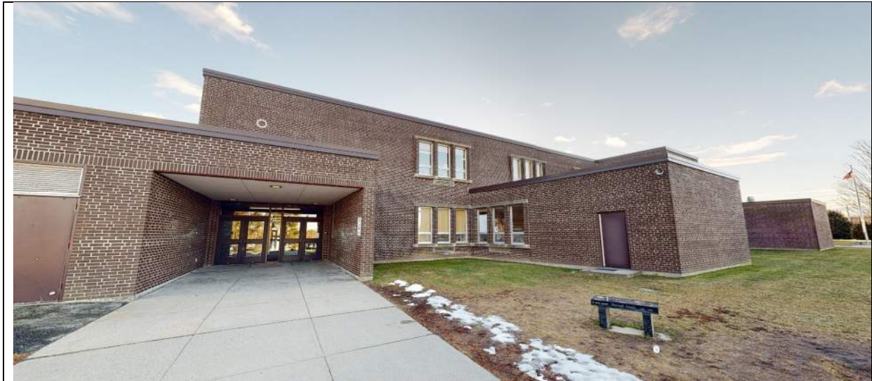
View of secondary entrance on north side of building.
