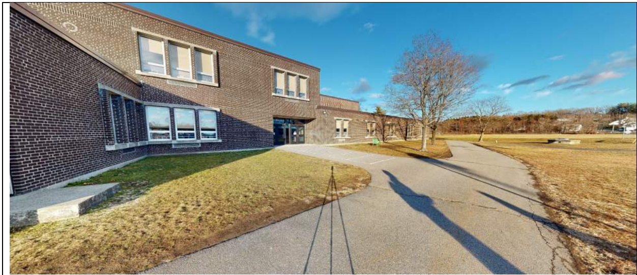
View at the southeast corner of the building, looking northeast.
