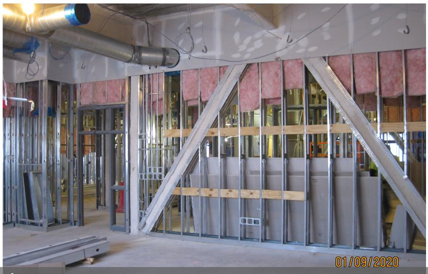
Interior Steel stud and structural bracing
