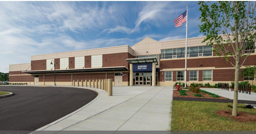
Exterior Precast concrete, brick masonry, and insulated metal wall panel at main entry
