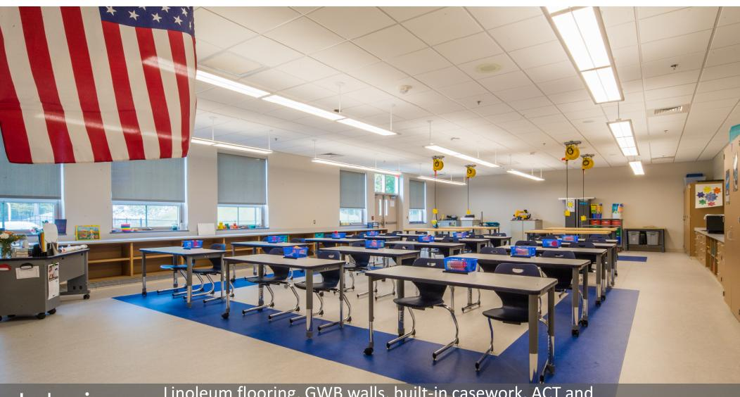
Linoleum flooring, GWB walls, built-in casework, ACT and indirect LED lighting at STEM and typical Classrooms
