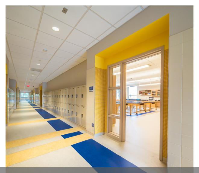
Hollow metal frames, corridor lockers, tile wall surface, and linoleum flooring
