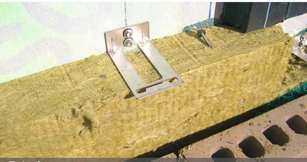
Exterior Brick masonry, fiber cement panel, and mineral wool insulation exterior wall
